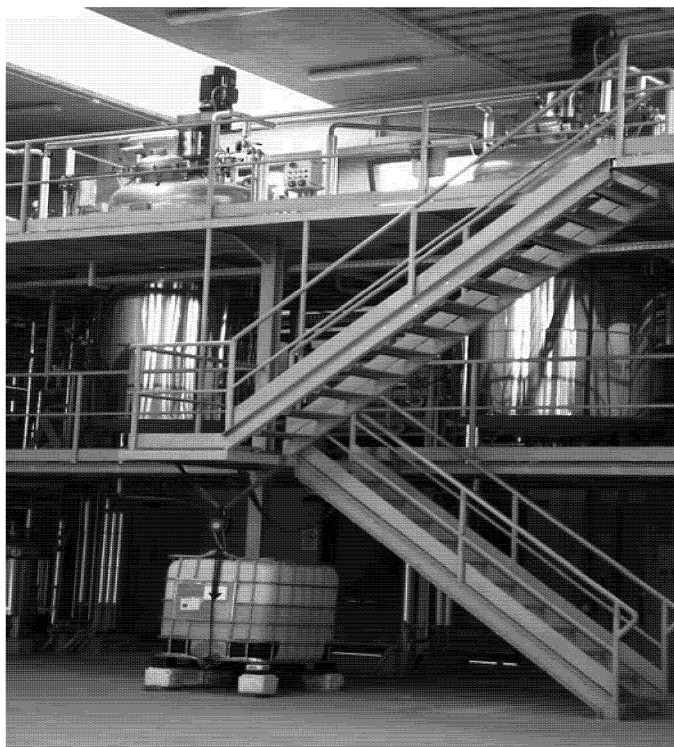
FIGURE 1 Bio & Geo Plant facility in Caserta
